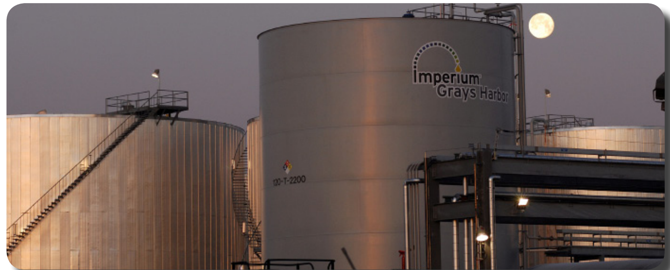
Imperium Renewables biodiesel production facility in the Grays Harbor IPZ
