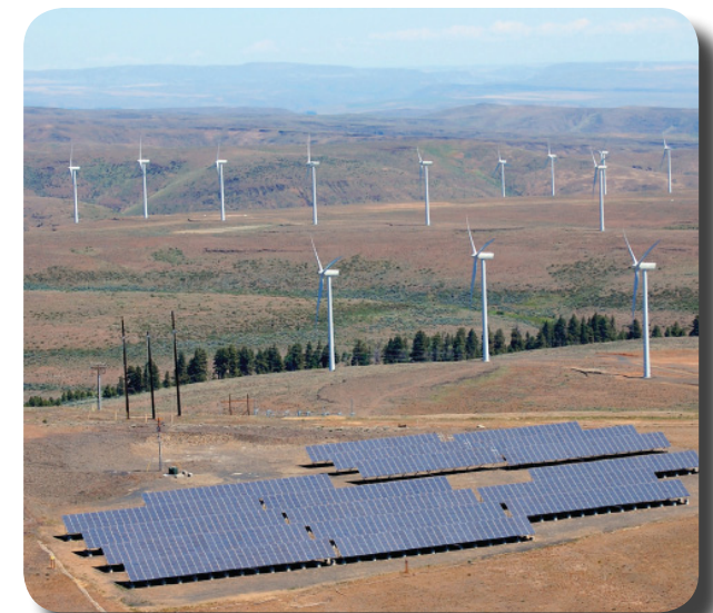
At 500Kw, the Wild Horse solar array is the Northwest's largest demonstration project of photovoltaic technology, which turns sunlight into electricity.
