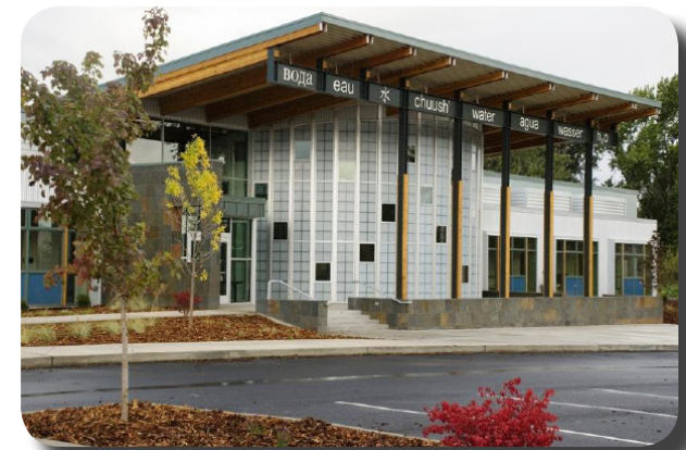
Water Center, Walla Walla Community College Campus
